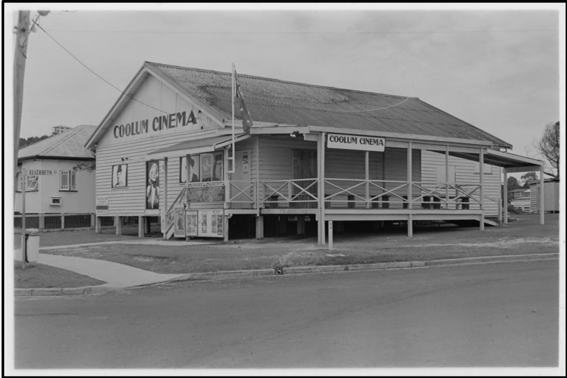
2.1.1 The Original Coolum Cinema (Circa. 1954) Now the Coolum Men's Shed Community Hall. (A separate building owned and maintained by the Coolum Men's Shed)
