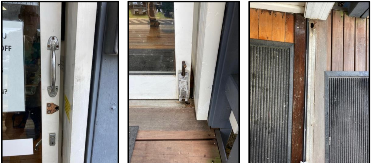
12.2 Community Hall at 26 Research St. (Men and Women's Sheds) Door Hardware Aged Condition of the Sliding Door Hardware.
